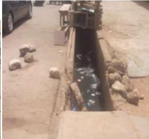
**Plate iv:** Clogged and blocked drainage with trash inside it **Plate v:** Broken drainage
